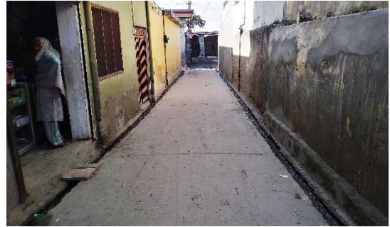
Street pavements/ sanitation work completed with the support of local government fund
